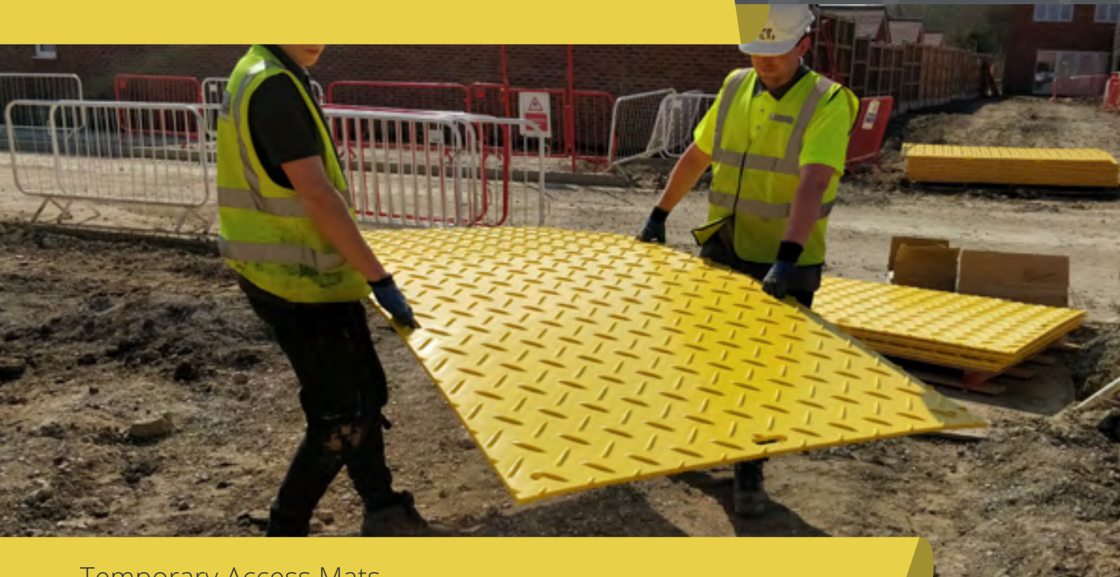
Temporary Access Mats
