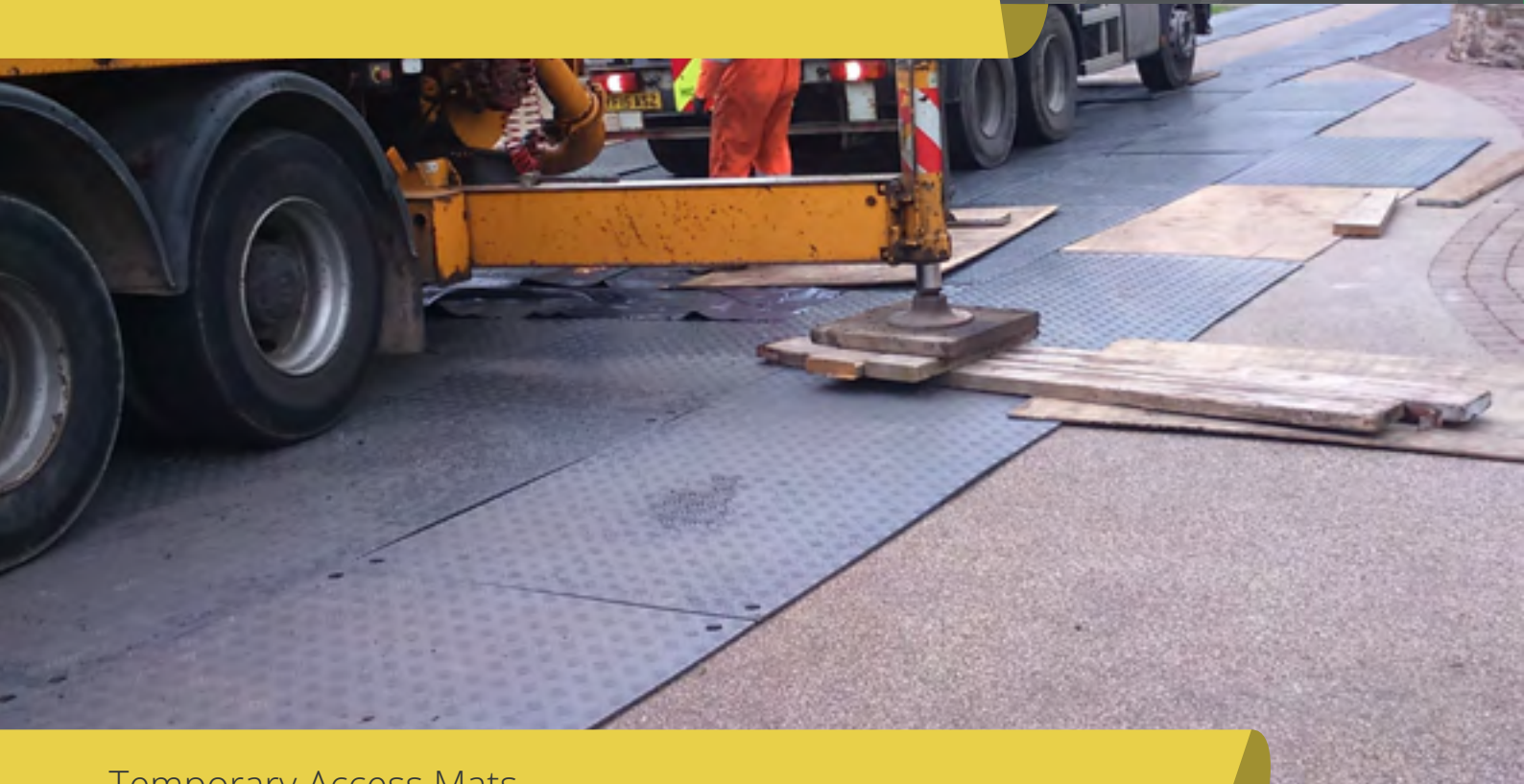
Temporary Access Mats
