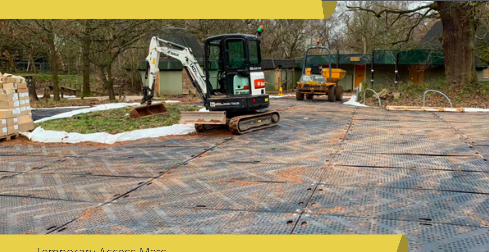
Temporary Access Mats
